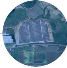
Inashiki Solar Park
